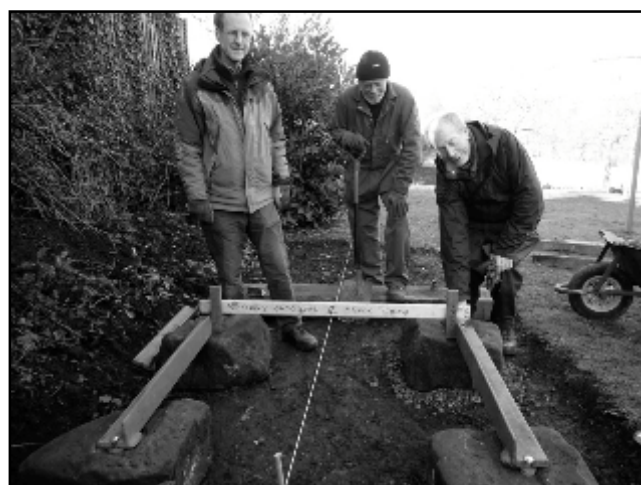
Track laying and wagon building
